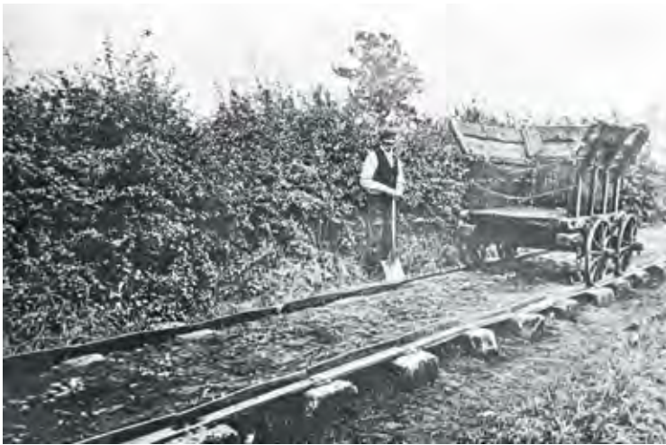
Fig. 2-17: Use of L shaped cast iron rails and stone blocks on the Denby Tramway-wagonway (Outram's Railroad) near Little Eaton, Derbyshire, England [28]
