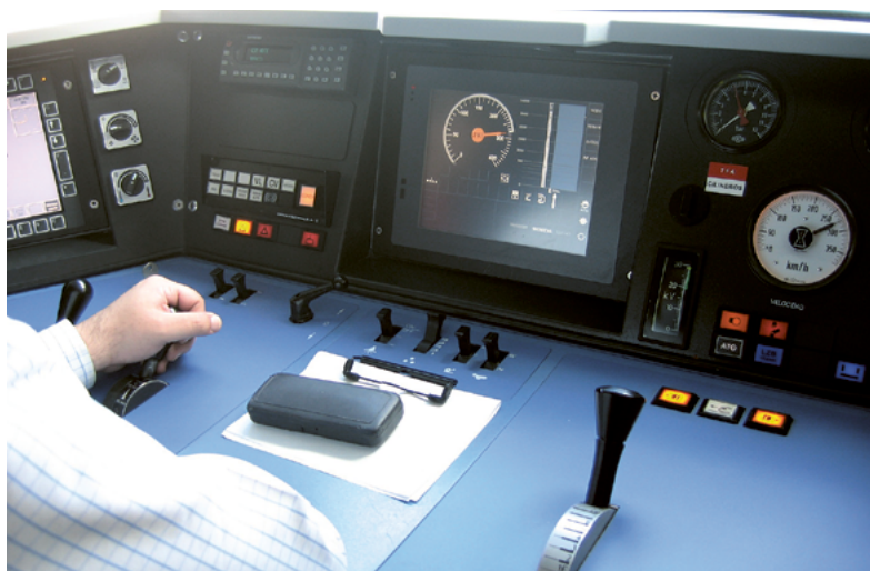
Figure 21-1: Typical DMI installation in cab, Class 102 train, Madrid (Siemens)
